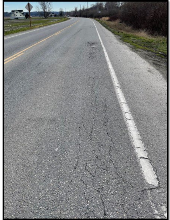
SOUTHBOUND LANE, MP 2.7
