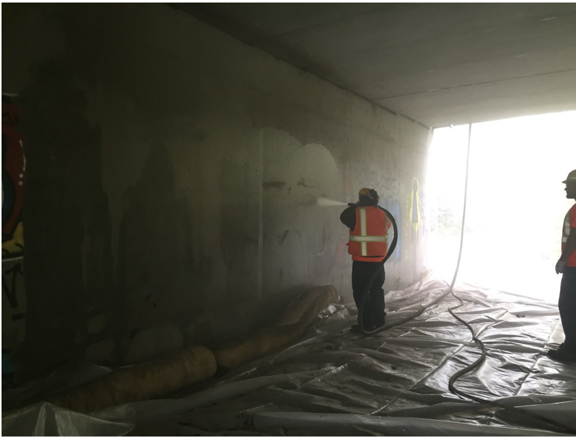
Straw wattles and plastic used to contain debris
