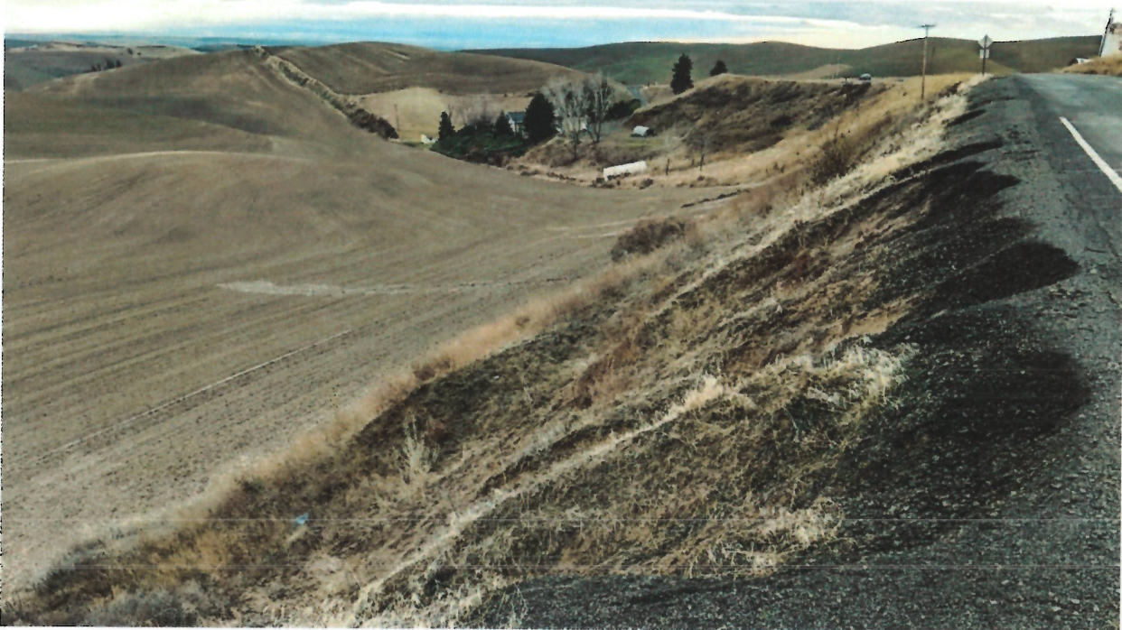
Approx. MP8.3 looking south.
